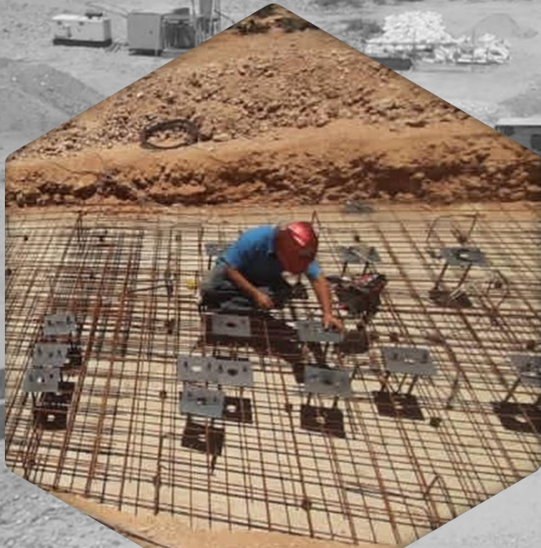
Dryer Foundation Work
